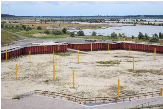
Construction area "New Harbour" in Großräschen (photo: R. Vigh/IOER)
